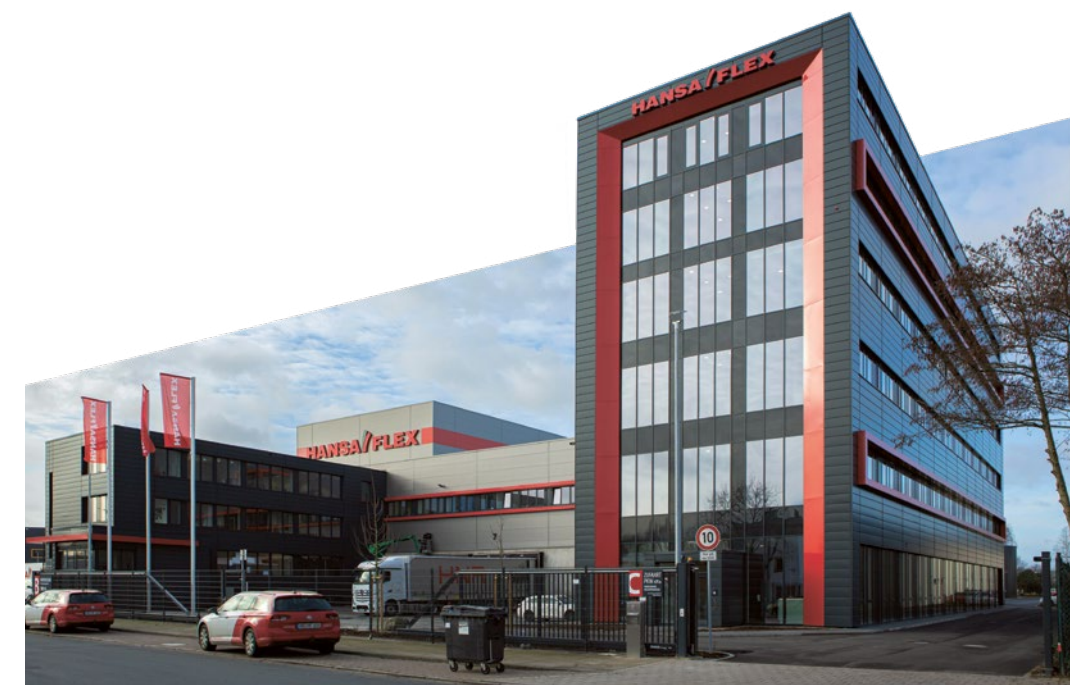
The large-scale project for the new logistics and production site with an investment volume of over 20 million euros creates more space for future company growth.
